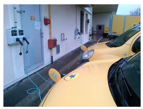
Example of Dynamic Power Management in Fleets. La Post France. Charging delivery EV's with the existing building power by intelligent and dynamic management system (in most cases no more power is available). This is implemented in multiple places, always the same solution.
