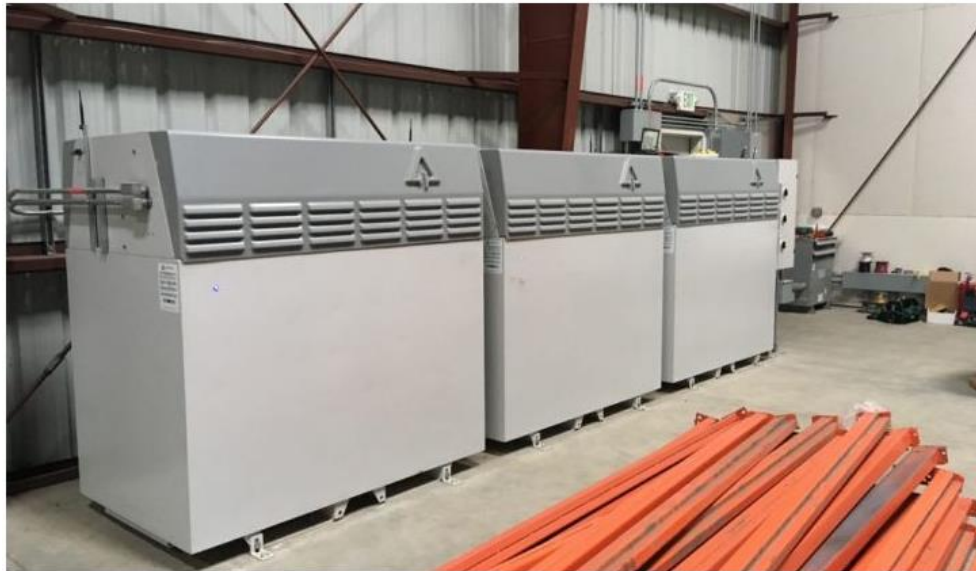
The Avalon flow batteries installed in a Santa Cruz microgrid contained a rented electrolyte to lower the project expense.
