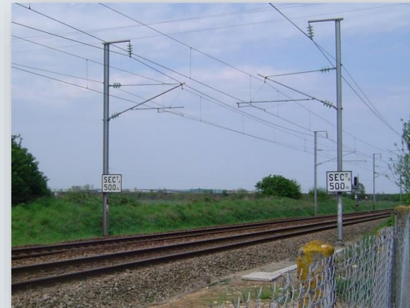
TGV Overhead Catenary System (France); AMTRAK AT station (USA)
