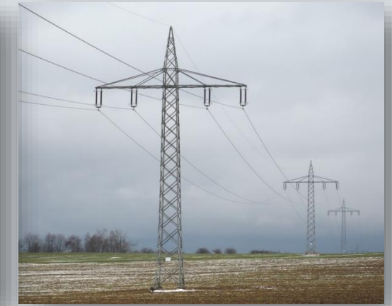
Deutsche Bahn, 1900's ~today at 15 kV AC ; Transmission grid at 110 kV AC 16.7 Hz
