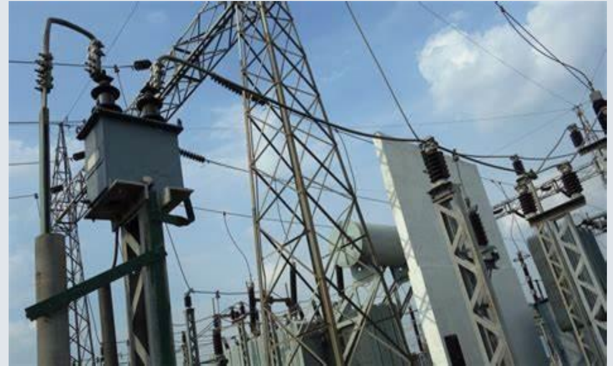
2x25 kV traction transformer (left) and outdoor switchgear (right) in Indian Railways
