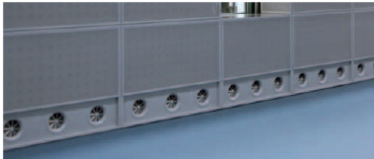
Lower chamber with swirl diffusers
